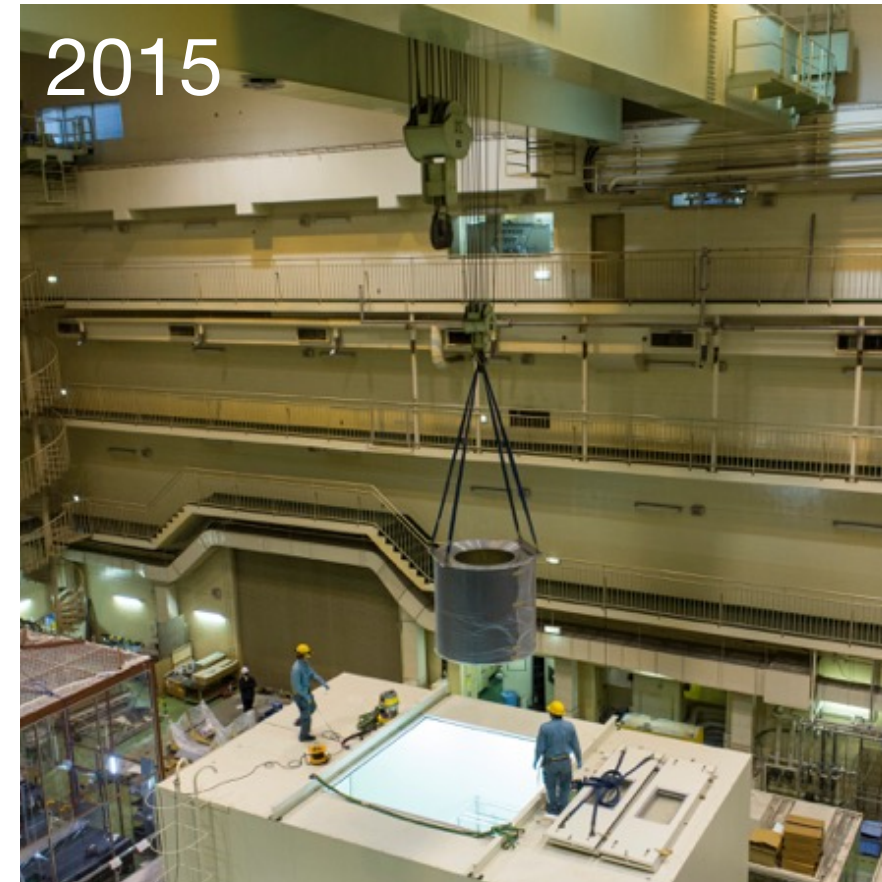
2015 Outer structure was transported to a KEK assembly hall, and set on a wire stringing cradle.
